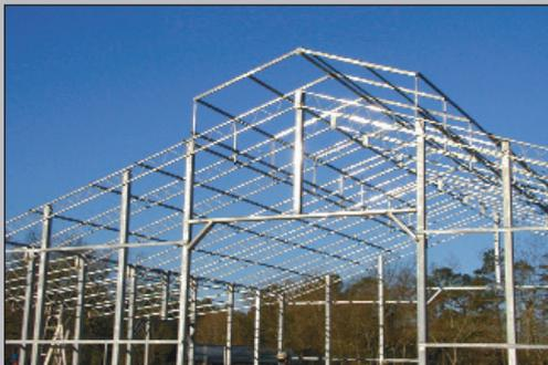
Hawthorne's SMARTFRAME Building System utilizes the V-truss design used on large buildings.
